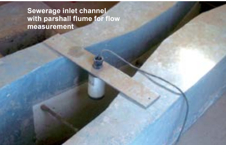
Waste water channel, with a rectangular flume for flow measurement
